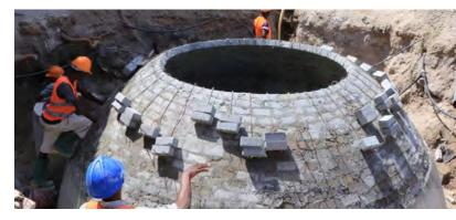
Biodgesters, like this one under construction at Mwananyamala Hospital in Tanzania, allow for the safe disposal of food waste and placentas, while generating biogas for use at the facility
